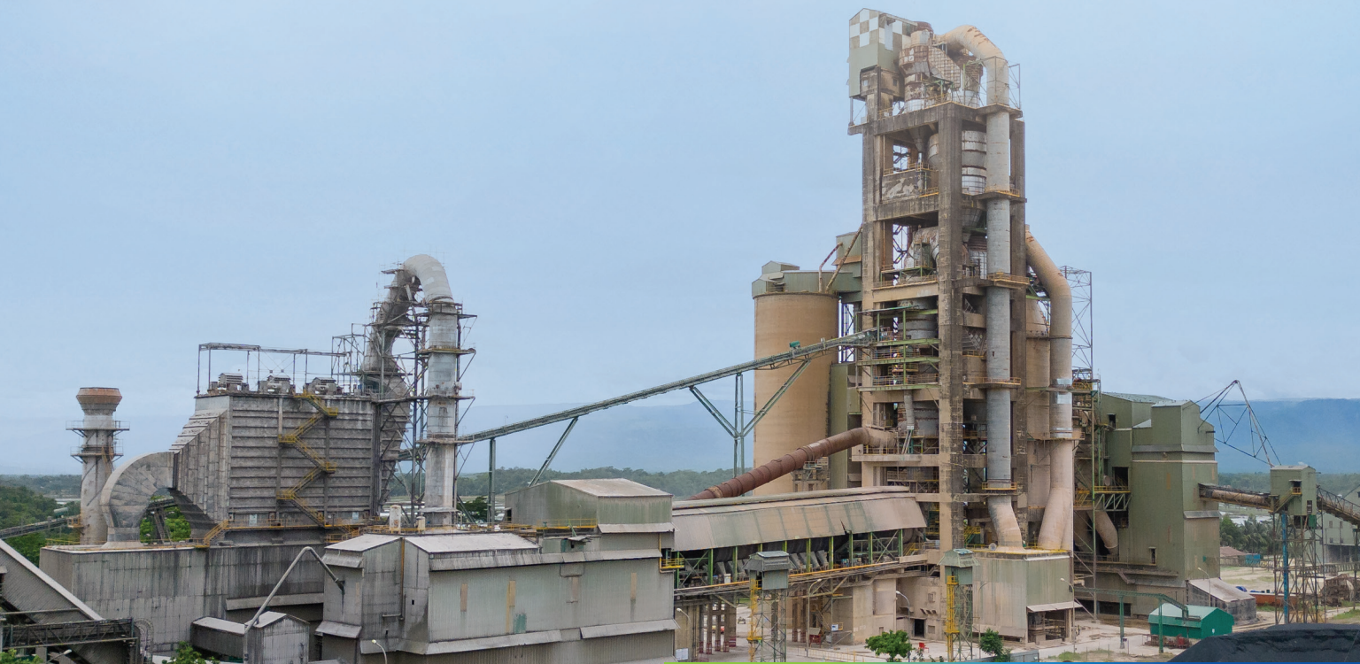
Surma Clinker Plant
